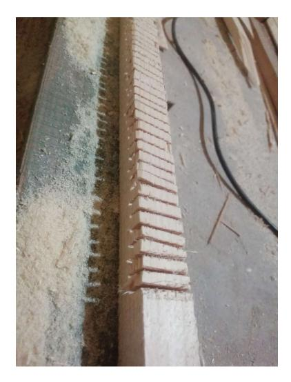
Use a handsaw to make them 5mm apart and for at least 30cm of the bending area. Saw roughly half way through the wood's thickness. Bend the stick towards the kerf and not the opposite way!
