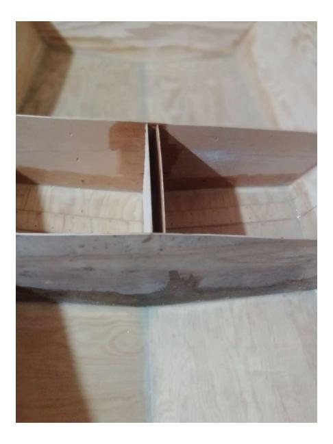
Pay particular attention when cutting the bulkheads out. The inside ones will obviously be the boat's bulkheads. The outside ones (the edges / frame) will be parts of your external temporary mold. And speaking of…let us see below.
