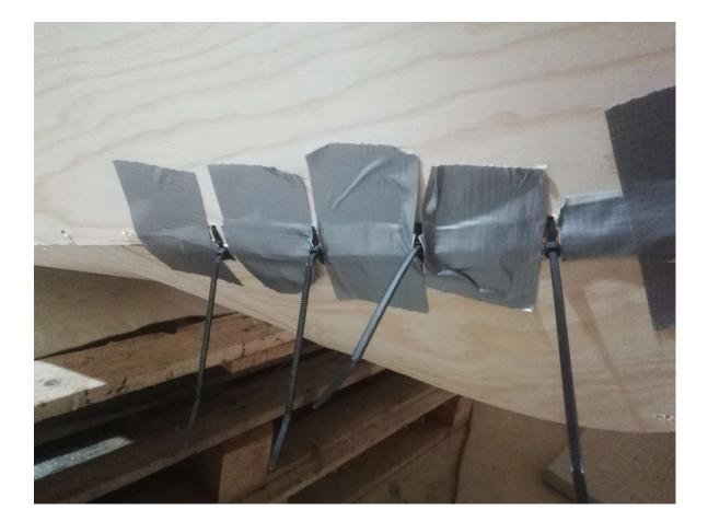
Remove all the cable ties except for the strictly needed ones. Your boat should be held together only by the glue.
